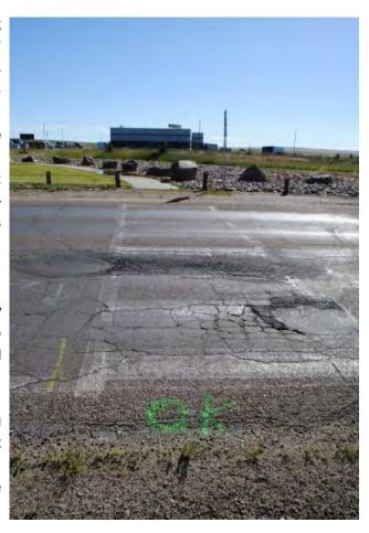
FIGURE 2 -- PAVEMENT DETERIORATION ON ANTELOPE DRIVE
